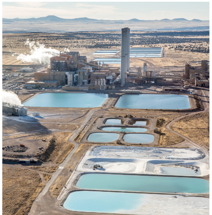
Tucson Electric Power facility, Springerville, AZ
