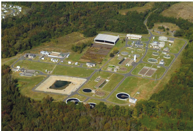
On-line ammonium sensors using new ion-selective electrode technology have enabled a North Carolina wastewater treatment plant to automatically control caustic dosing for greatly improved process performance.
