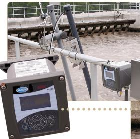
The staff at Rock Creek WWTP has seen a significant reduction in energy costs after installing the LDO probes and Hach controllers. Automating aeration based on current DO levels has brought an estimated power cost savings of approximately \$3,500 per year per basin, or a total of about \$14,000 per year if all four basins are operated.
