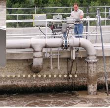
controllers on the basins, or they can be adjusted from the plant SCADA. "We programmed all four controllers to turn the blowers on and off at a specific DO level," Daniel said.
